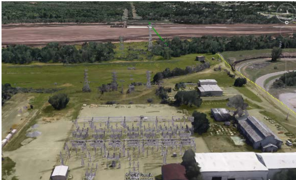
Figure 5: Looking South At Prattville Creek Outlet, Google Earth 2016, Green/Yellow Line Represents Location Of The 8.8 Mile Dam Alternative Site
