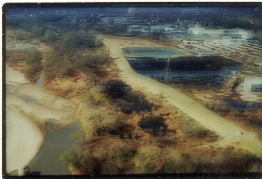
Figure 10: Sand Springs Petrochemical Site Photograph Prior To Excavation of Sludge, Looking west
